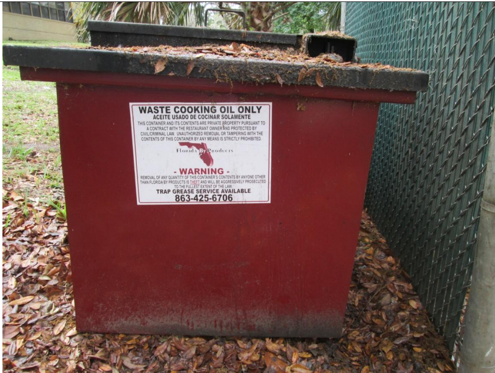
Photograph 7: Kinne University Center, 310 Gallon Kitchen Grease AST
