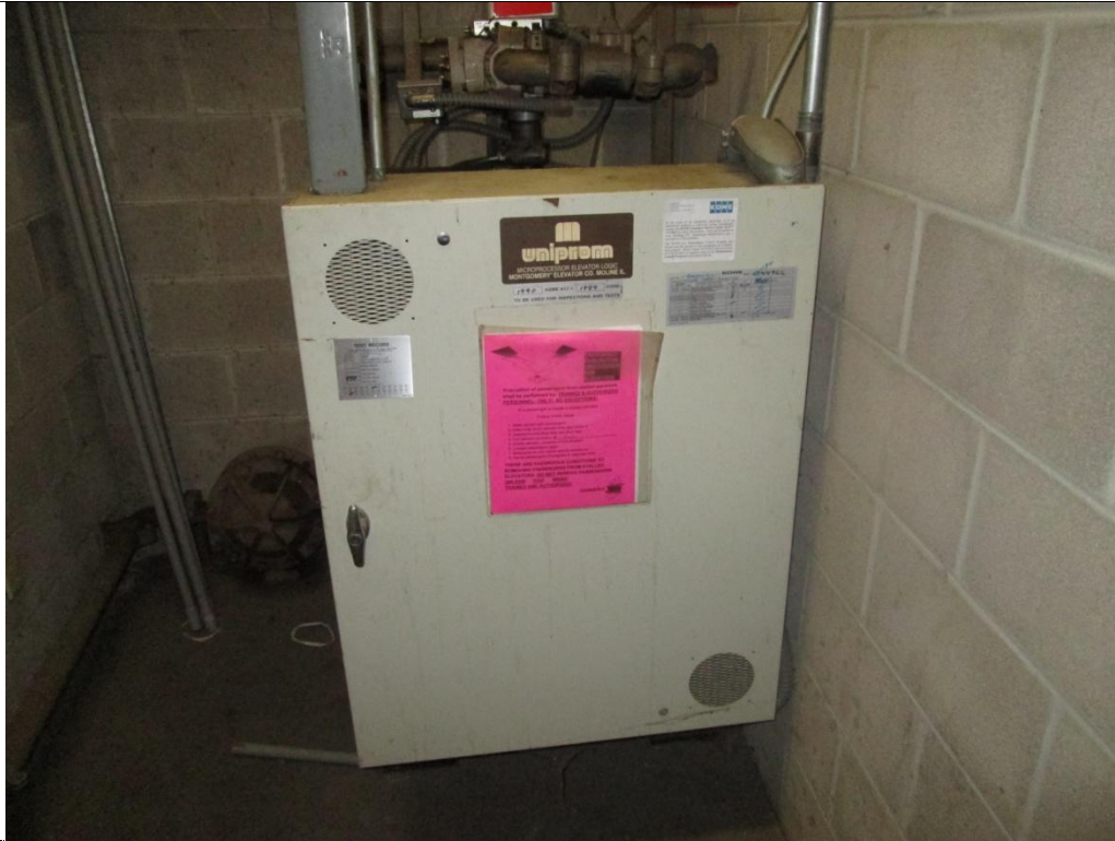
Photograph 3: Davis Student Commons, 90 Gallon Reservoir Hydraulic Elevator
