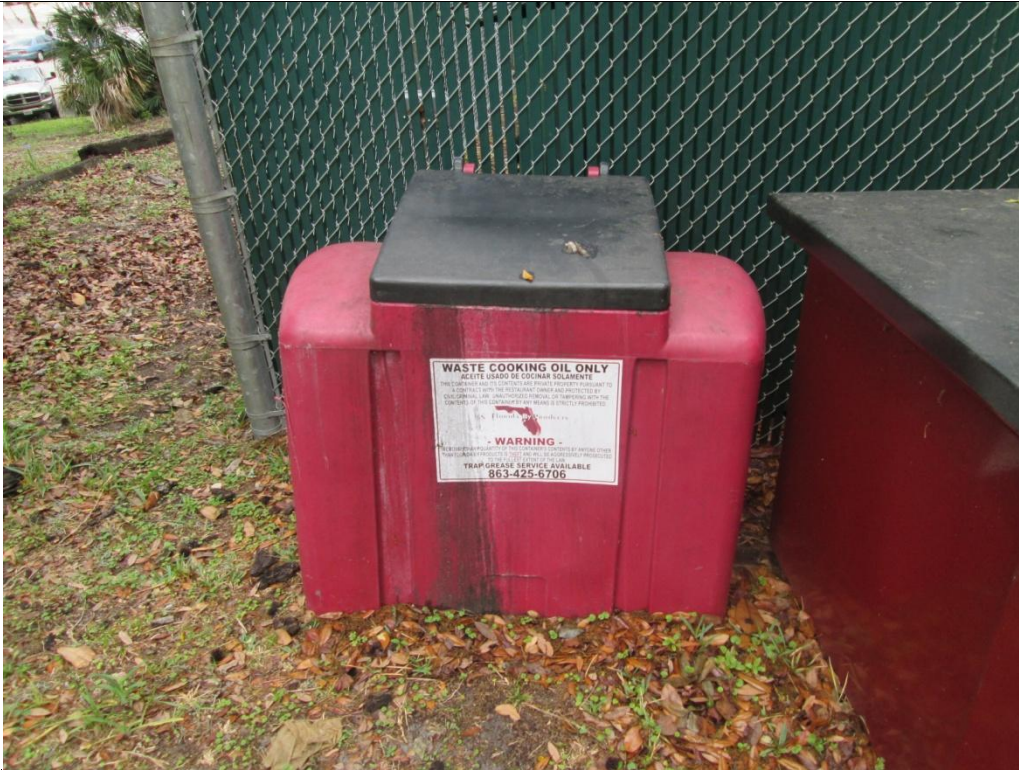
Photograph 5: Kinne University Center, 125 Gallon Kitchen Grease AST
